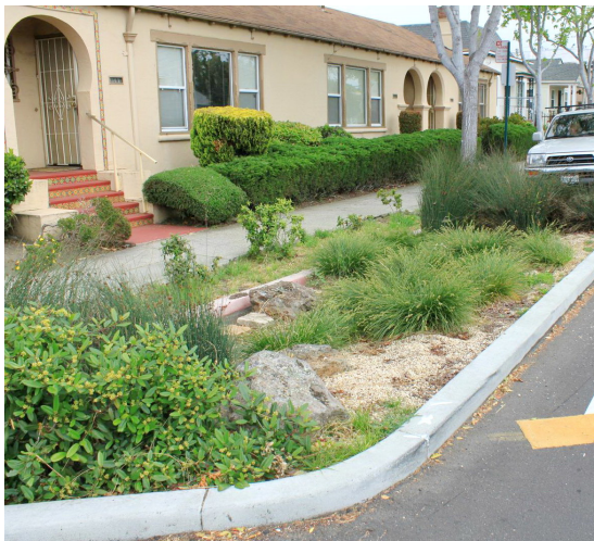
Stormwater swale interspersed with on-street parkingW
