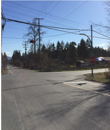
Key intersection of Bell McKinnon Road and Herd Road
