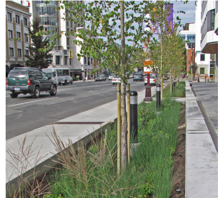
An urban stormwater swale with street trees
