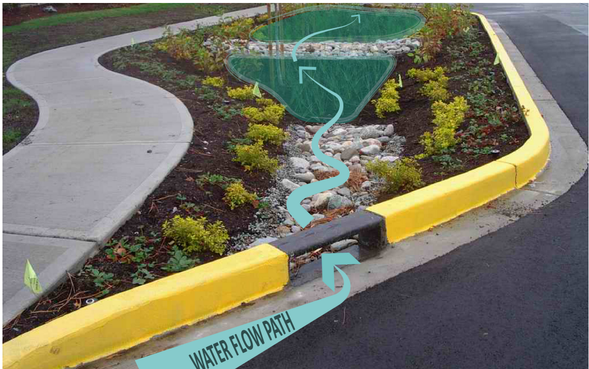
Stormwater flow path into on-street raingarden
