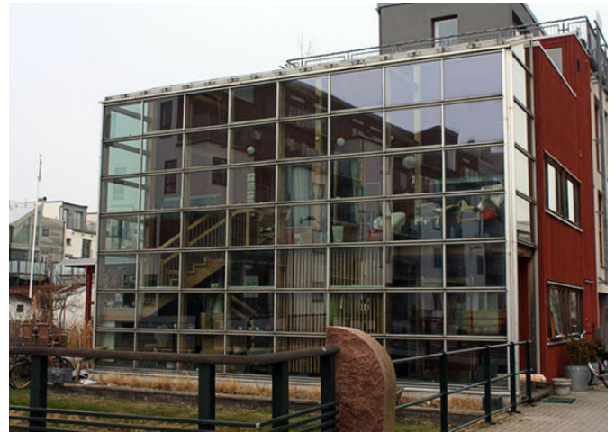
Example of a light industrial building integrated into a predominantly residential area
