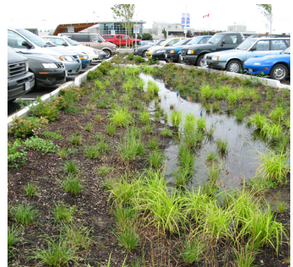
An on-site raingarden receiving parking lot run-off
