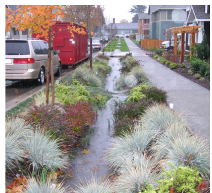
A suburban stormwater swale
