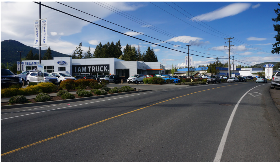
Despite road improvement in some locations, on-site pedestrian and cycling facilities are largely absent in the area
