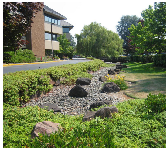
A landscape-based stormwater detention area
