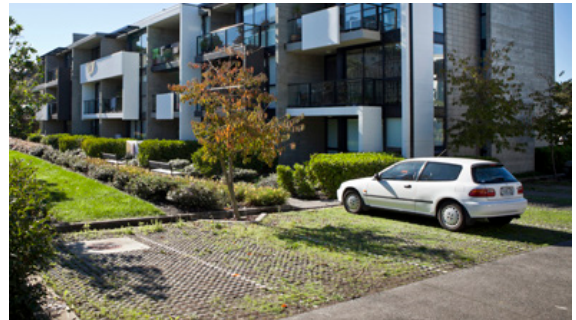
Permeable paving in a surface parking lot
