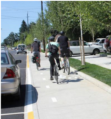
A raised separated bicycle facility
