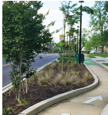
A physically separated bicycle facility
