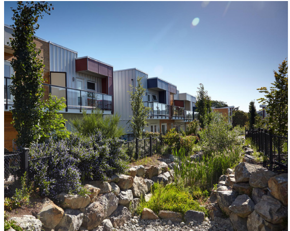
Large landscape-based stormwater facility in a multifamily development
